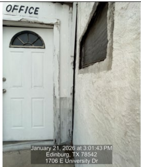
Separation of Masonry
