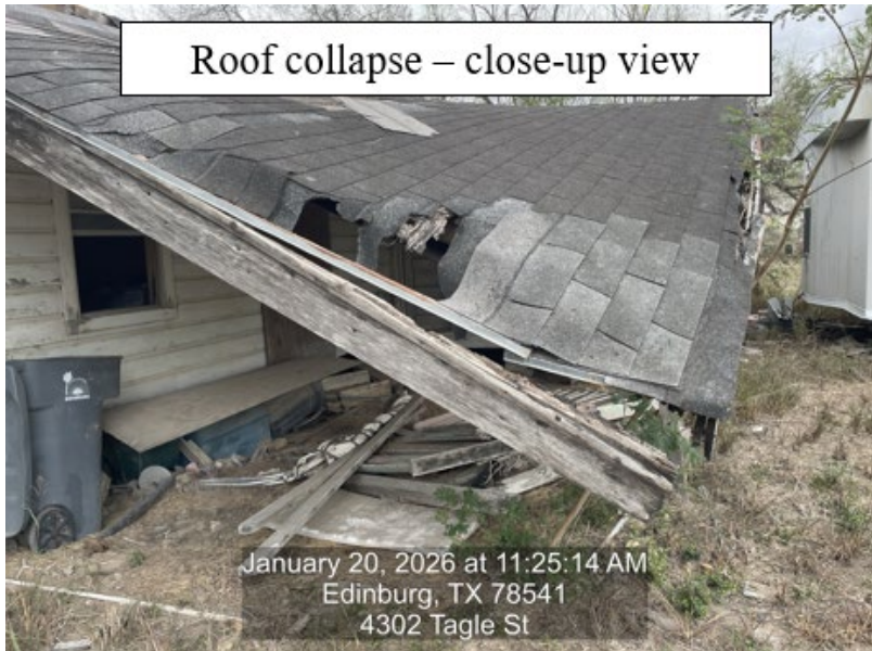
Roof sections separating – close-up view
